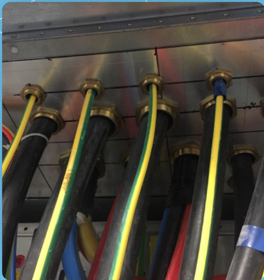
2500Amp MV Panels & Substations Many Different Location
