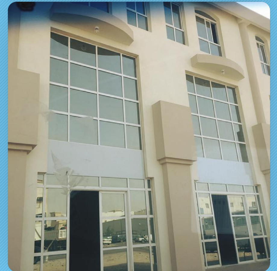
(G+2) Commercial Building Industrial Area - 2016
