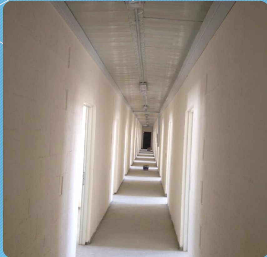
Labour Camp 1000 Rooms Client (Sodexo ) Location: Al-Khore - 2016
